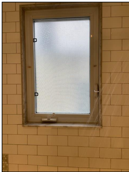
Window in shower enclosure
